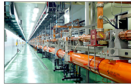
Pohang High Energy Radiation Facility with 2.5 GeV e-linac
